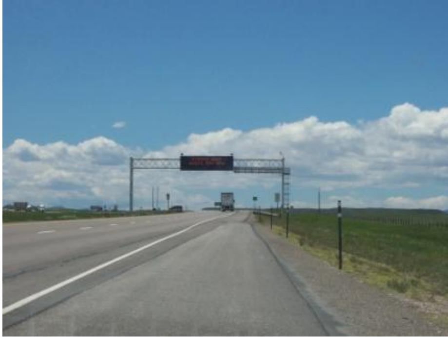
Figure 14: Photo. Three Line, Overhead Mounted DMS on I-80
