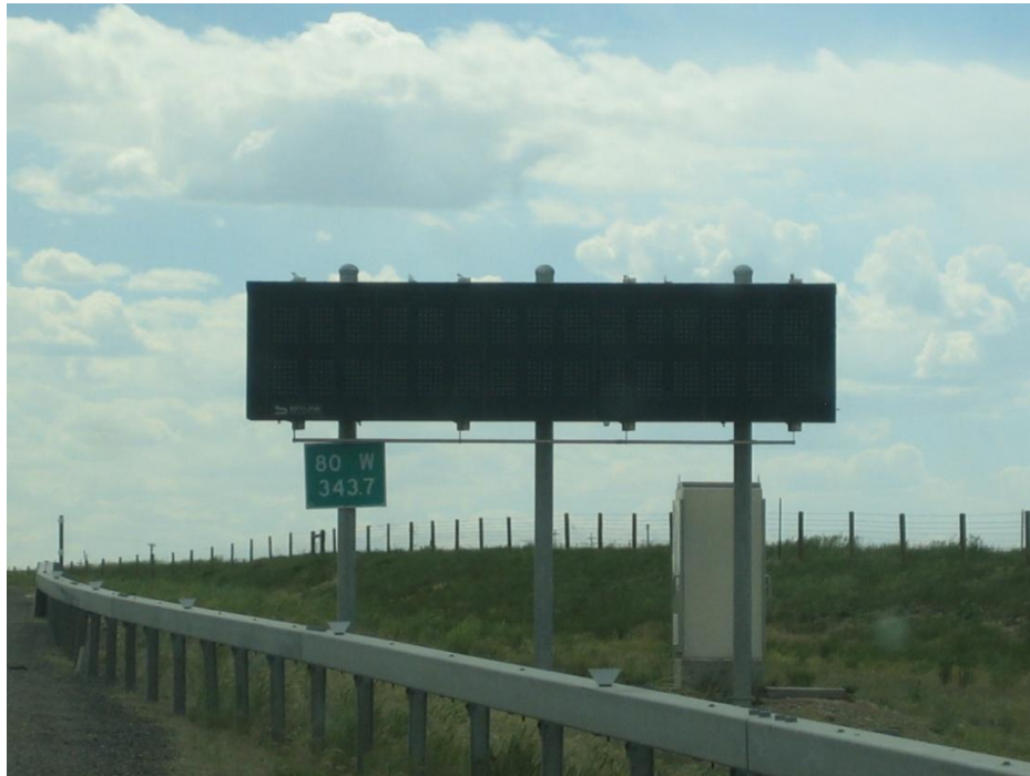
Figure 13: Photo. Two Line, Side Mounted DMS on I-80
