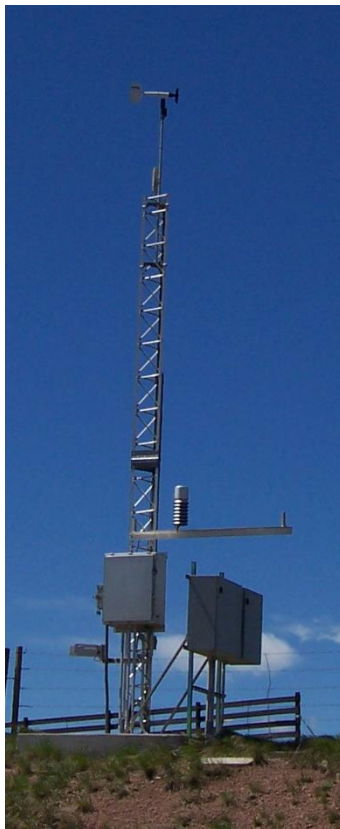
Figure 10: Photo. RWIS Station on I-80
